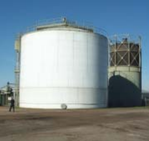
Anaerobic digesters (left) and a covered anaerobic pond.
