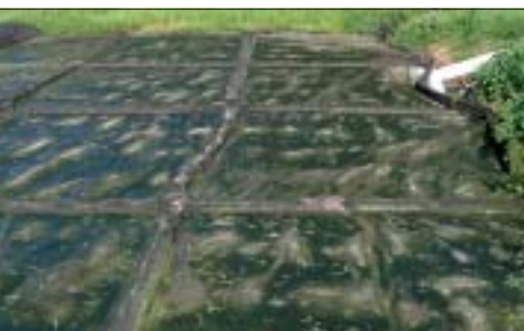
This anaerobic pond has an impermeable cover which greatly reduces odour emissions.
