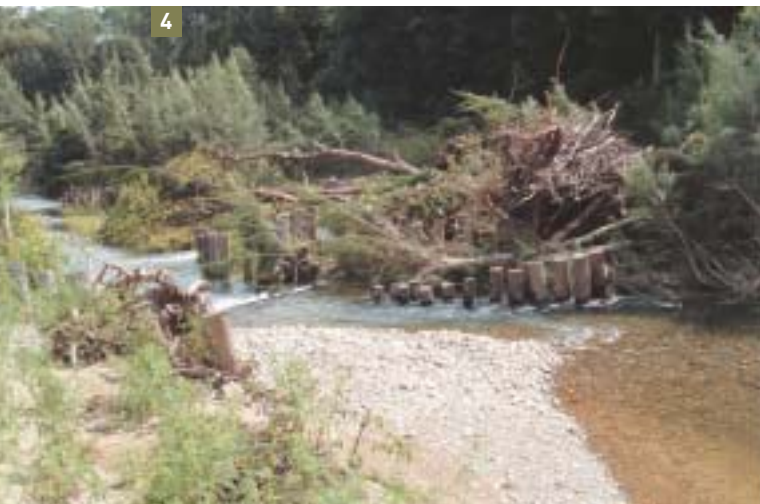
4. Site Two — view from upstream. Elevation of upstream water levels has promoted gravel deposition and riffle formation upstream of ELS.
