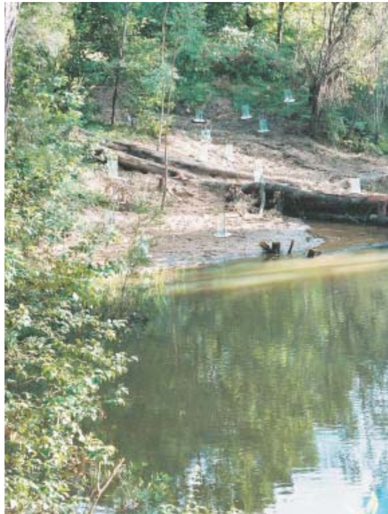
Photo 3. Constructed bed control log structure — Stockyard Creek, NSW.
