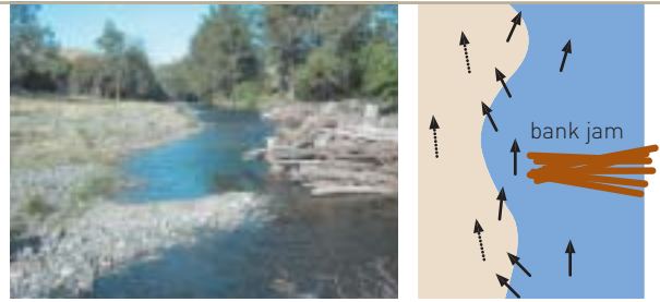
Figure 5. This constructed deflector jam (DFJ) extending into the channel in the Williams River caused scalloping of the edge of the gravel bar across the channel, enhancing the surface area for lateral hydrological exchange, represented by arrows in the schematic diagram.
